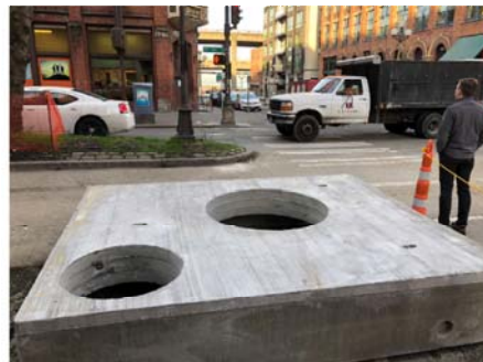
Lid for water valve vault.
