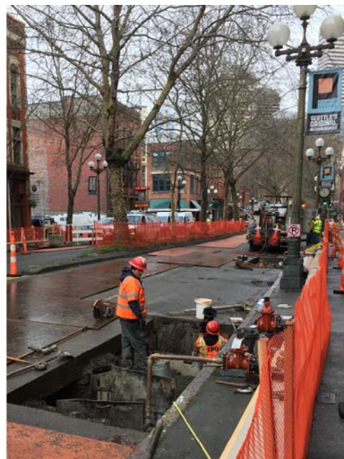
Seattle Public Utilities transferring customers' service to the temporary water main
