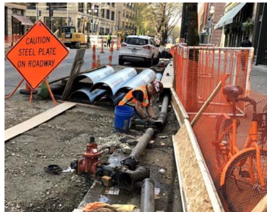
Dismantling temporary water main on 1st Ave S
