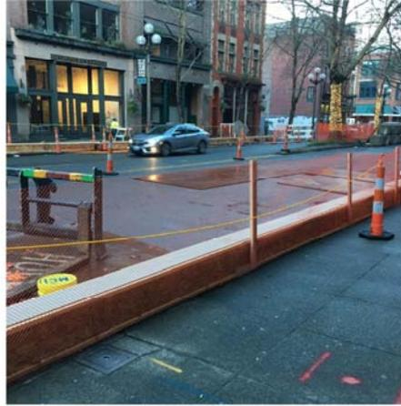
Temporary water line installed on 1st Ave S and protected by wooden casing
